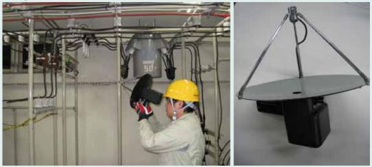
which can measure supersonic wave generated due to insulation deterioration
