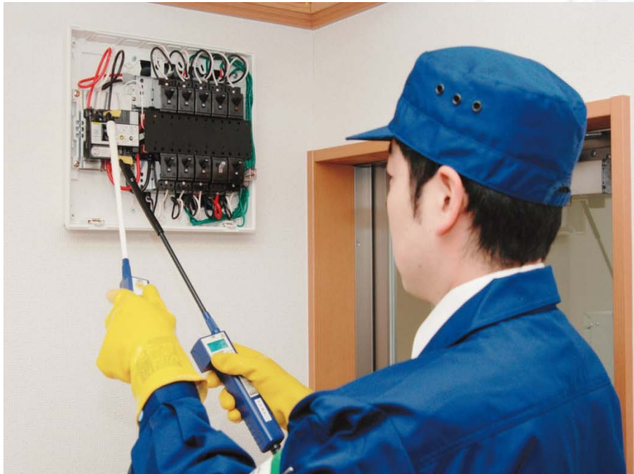
Insulation resistance measurement
