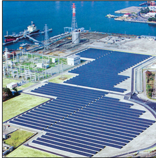
Example of large- scale installation
