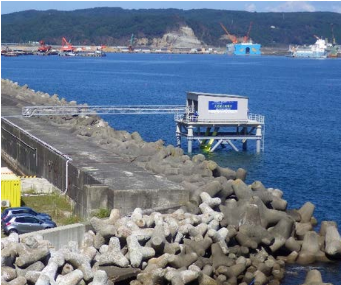
Example of a wave-power generation installation
