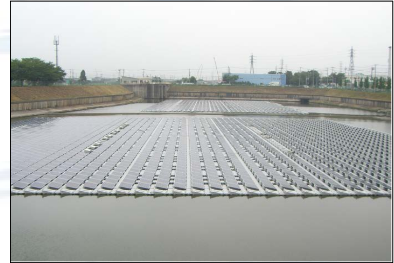
Example of installation on body of water
