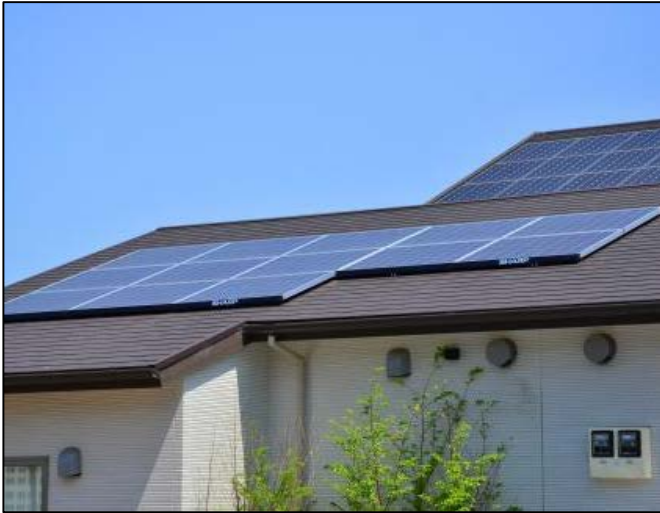
Example of installation on home rooftops
