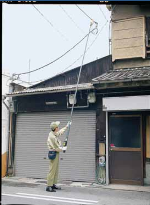
Leakage current measurement at a customer's site where an ordinary measurement cannot be carried out readily.
