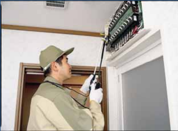
Insulation resistance being measured with a distribution switchboard
