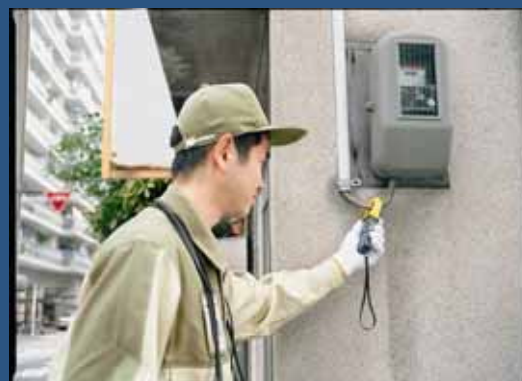
Verification of insulating state through leakage current measurement (The acceptable leakage current value should be 1 mA or less.)
