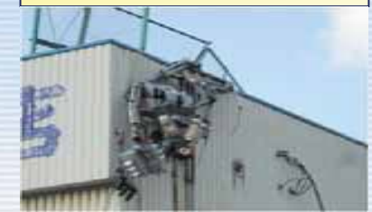
A transformer within a high voltage receiving unit
