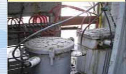
A transformer within a high voltage receiving unit
