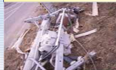
A high voltage receiving unit buried in the debris
