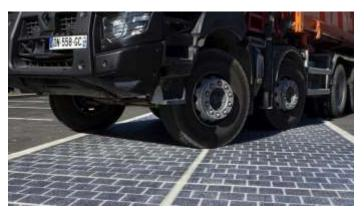
The photovoltaic road, a world first, was launched in France in October 2016. Photovoltaic cells, in the form of tiles, are glued on roads or in car parks.
